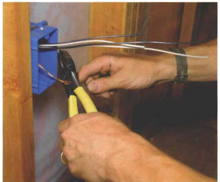
Special side-cut pliers dimple-crimp the grounding connector.
