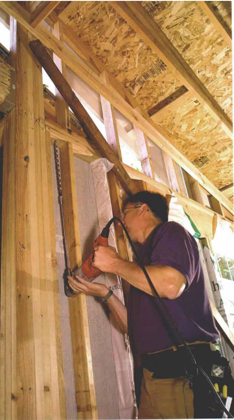
Going 'round the bend. After drilling intersecting holes, the author strips the cable to expose an easily maneuvered single wire. He works this wire around the turn and uses it to pull the cable.
