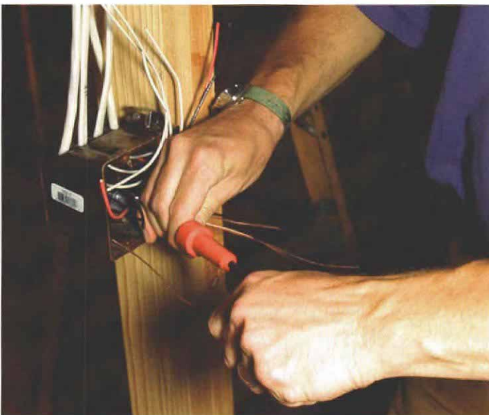
Wire-nut driver ensures tight connection.
