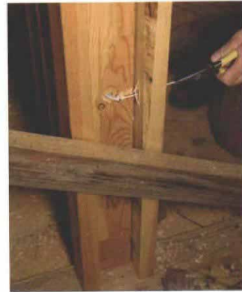
Going 'round the bend. After drilling intersecting holes, the author strips the cable to expose an easily maneuvered single wire. He works this wire around the turn and uses it to pull the cable.
