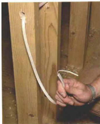
Going 'round the bend. After drilling intersecting holes, the author strips the cable to expose an easily maneuvered single wire. He works this wire around the turn and uses it to pull the cable.
